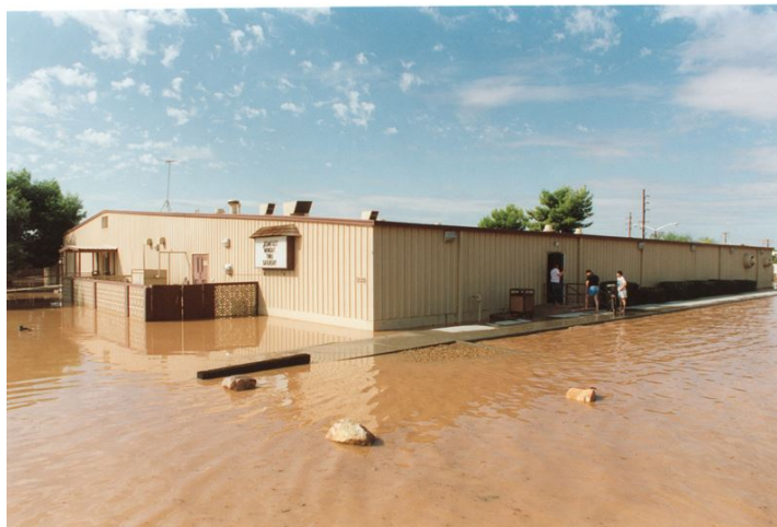
Flooded Base Bowling Alley, 20 October 1992
