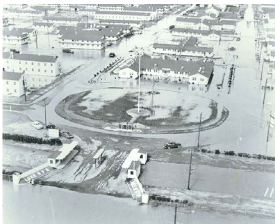
Flooded Front Gate
